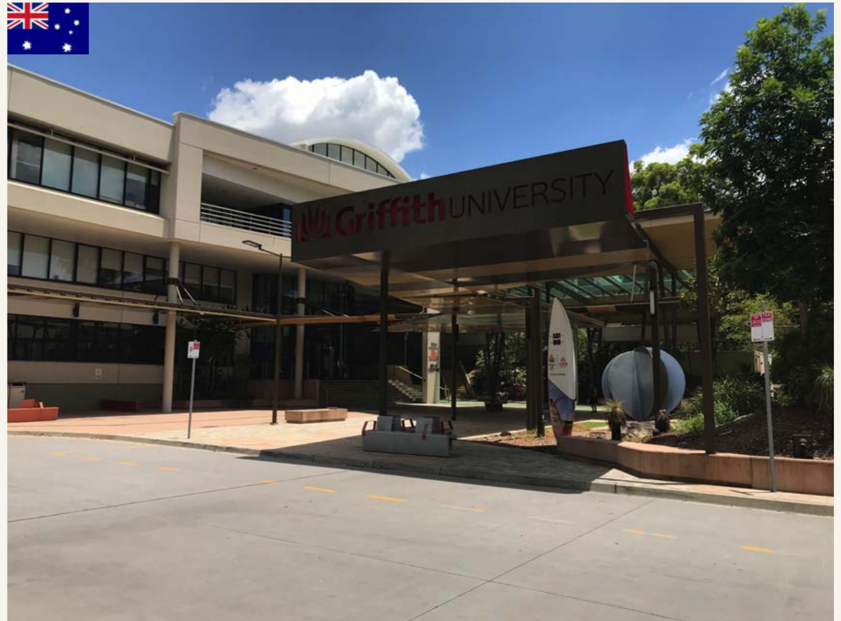
Australia, Griffith University, SVG 4300kvar A very big campus with many transformers, some challenge SVG installations are 200M from coast with high corrosion by IP54 outdoor SVG
