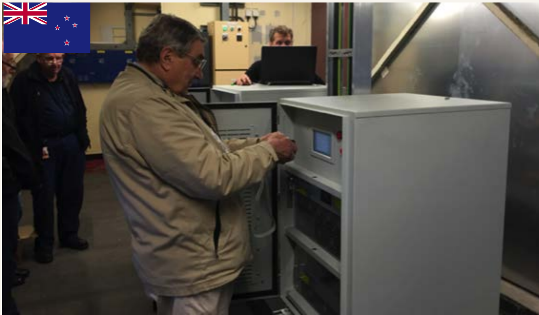
New Zealand, Parliament Library, SVG 200kvar John Fulton was taking photo for SVG performance, because he was surprised at the consistent Cos fi 0.99 by SVG
